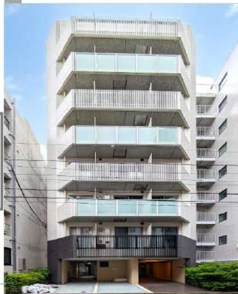
TRESTELLA RESIDENCE IRIYA
